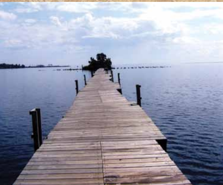
3 RD Washburn Pier Tim Van Blarcom—Viroqua, Wisconsin
